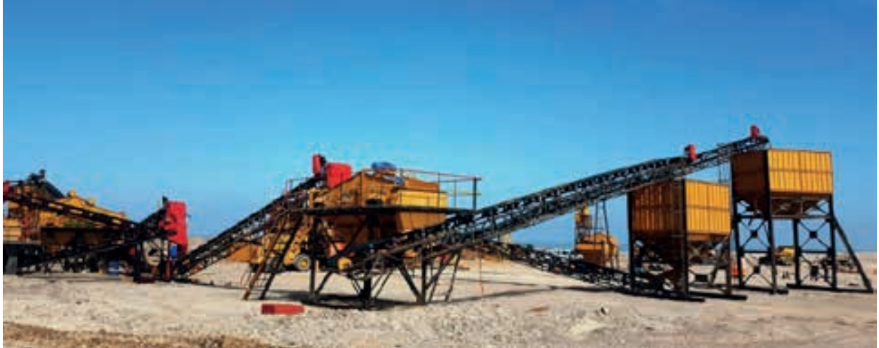
NNDC processing plant, April 2016
