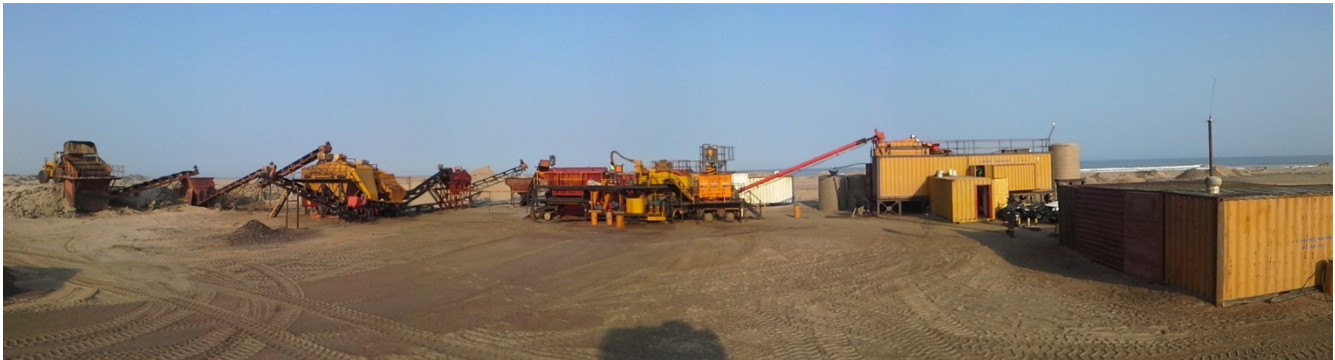
Fig 60: Panorama View of Processing Plant
