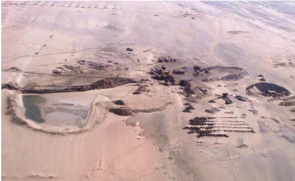
Fig 63: Aerial View of Processing Plant, Waste Dump, Tailings Dam, Feed Stockpiles
