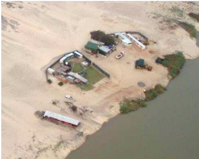
Fig 62: Aerial View of Admin/Accommodation/Workshop Facilities
