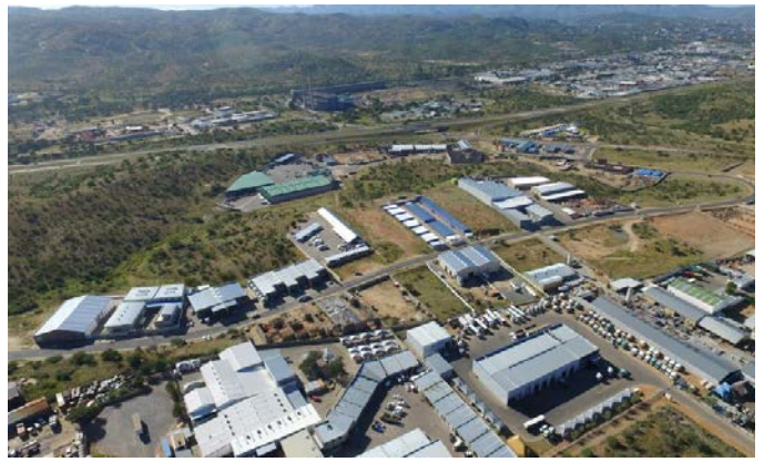
Figure 22: Lafrenz Industrial Park Extension 1 (After)
